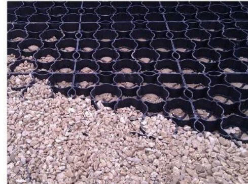
Ground reinforcement grid
